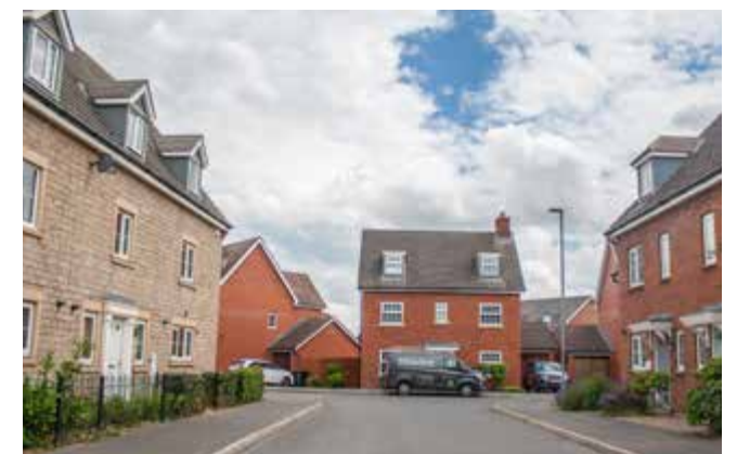
Residential development in Calverton
